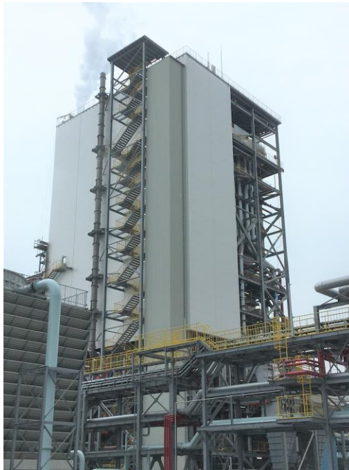
Figure-1 A whole view of biomass power plant after operation (Project 02)
