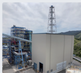
Waste-to-energy boiler (No. 5 boiler) at Iwaki Daio Paper
